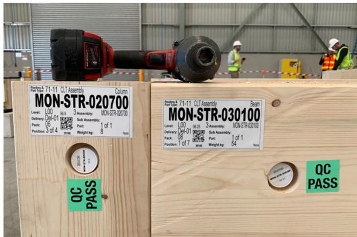
Figure 3. Assembled and tagged timber components
